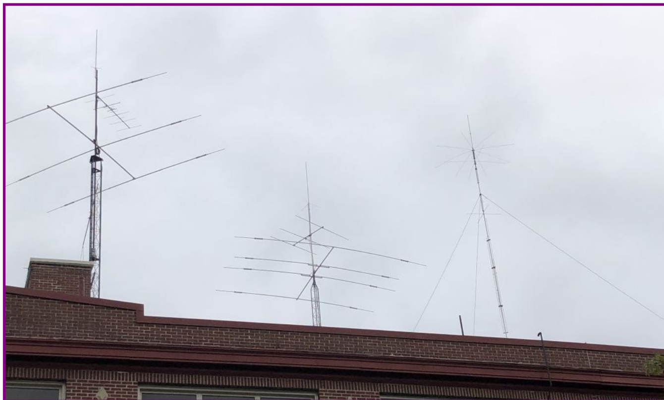
Beams on towers, R9 Vertical, and other station antennas on roof
