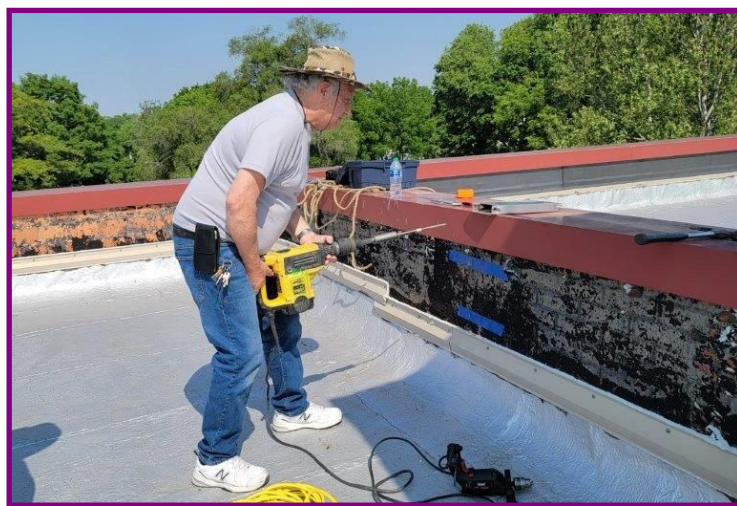
Drilling Mounting Holes for R9 Tilt Bracket
