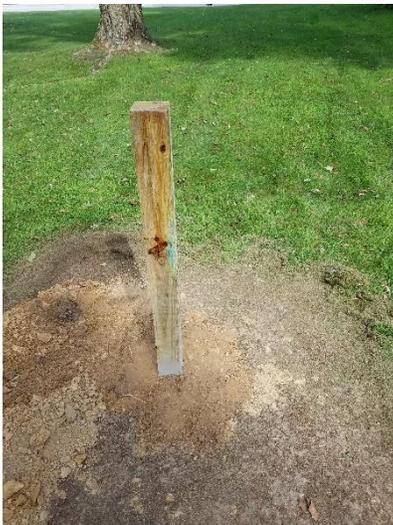
After I got the backfill in, I used 2 levels just to make sure that the post was level and plum. After all, I didn't want to go to all of this work and have my antenna tilting over like the Leaning Tower of Pisa!
