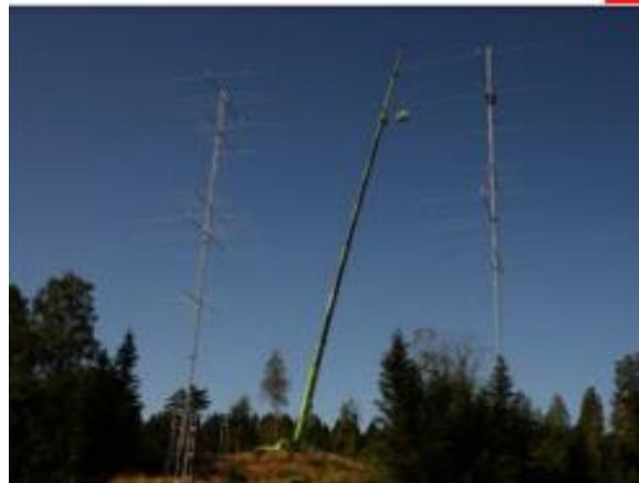
*Figure 2 The two 56-meter towers, and E77DX installing the 50m beam.*
