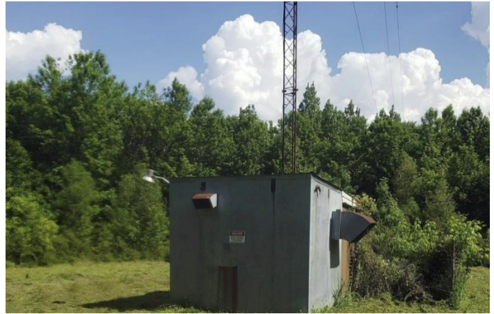
WJLX AM transmitter site, photo "taken within the last two years" (Radio World)
