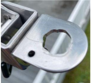
The clamp with the hold bored out to 5/8" (click to enlarge)
