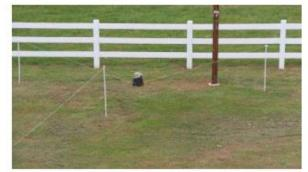
Here are three Beverages (in different directions) coming to a common feed point. A plastic "bucket" makes a weather-proof cover for the three Beverage feedpoint.
