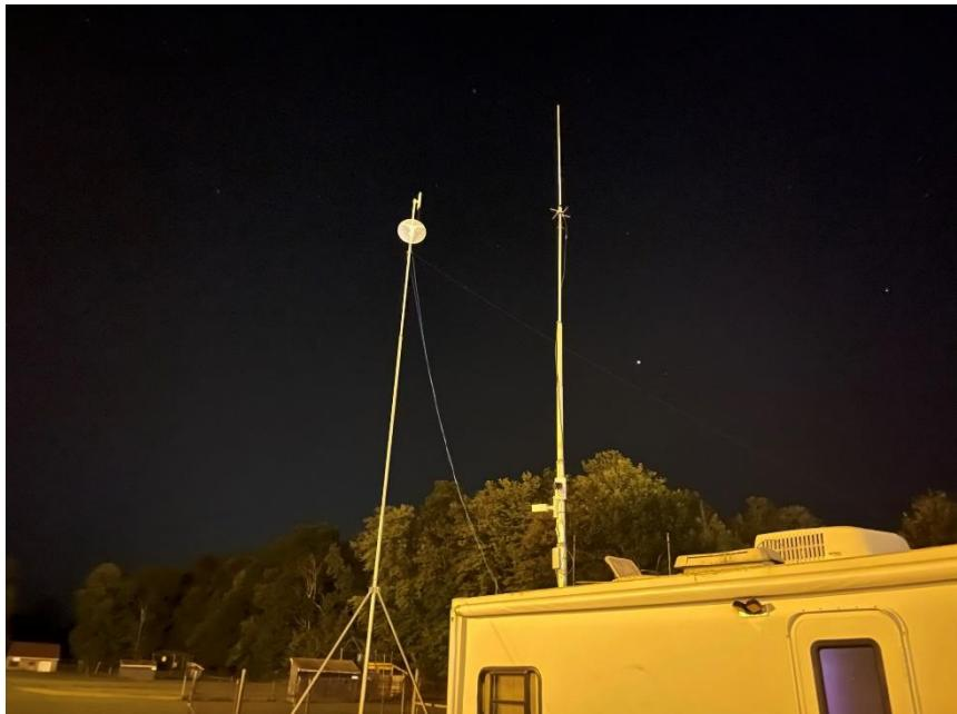
We also run an IP camera system and a VoIP telephone system - using microwave links - to help provide the Sheriff's Office and the Fair Office with better visibility into traffic and parking conditions.
