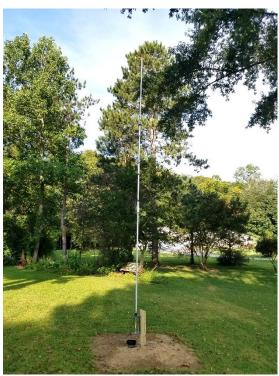
Wow.. once again, I had a tough time with the choke, but I finally got it and with the connector mounted I'm ready to connect to the radio. Since I already have another antenna just for 75/80-meters, I have to insert a coaxial switch so that I can switch between the two antennas. Got all of that mounted and a new jumper between the switch and SWR bridge. I'm now ready to test the antenna.
